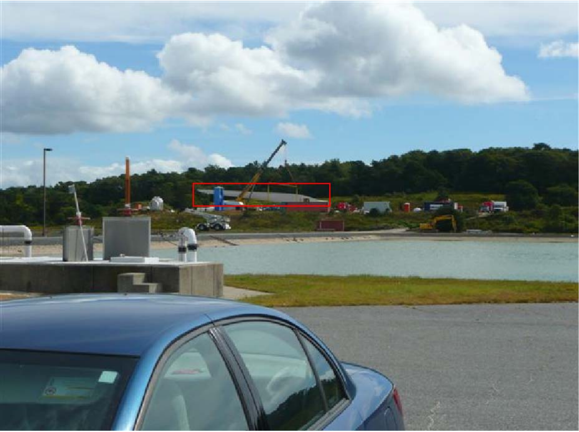
View from Treatment Plant 900 feet away – Crane lifting a blade
